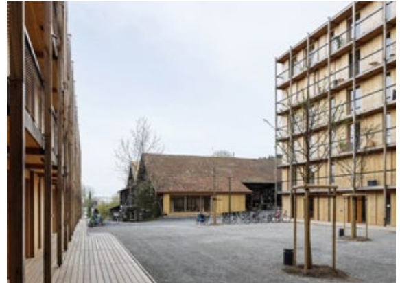
Hagmannareal Affordable Housing, Winterthur, Switzerland
