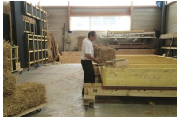
Prefabricated sustainable social housing, Nogent-le-Retou, France
