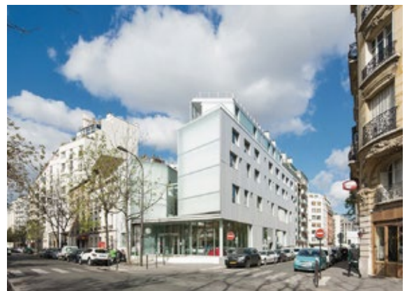
Mixed use building with social housing, Paris, France
