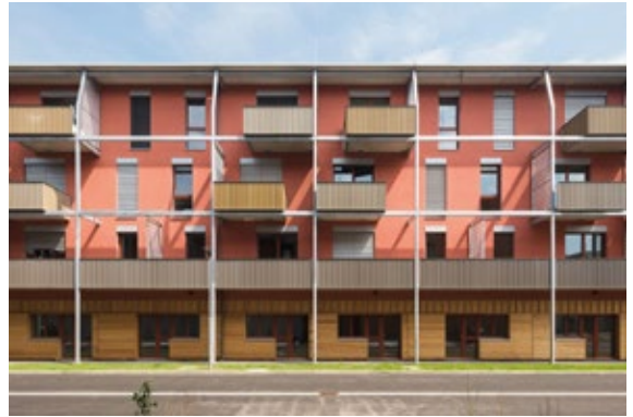
Multifunctional building – temporary rapid housing, Vienna, Austria
